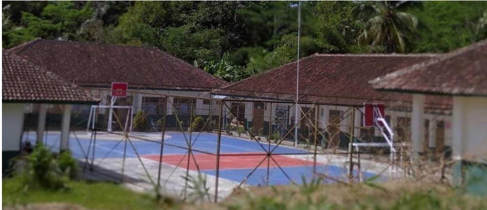
Picture 10. The condition of building of SMK Yapim
