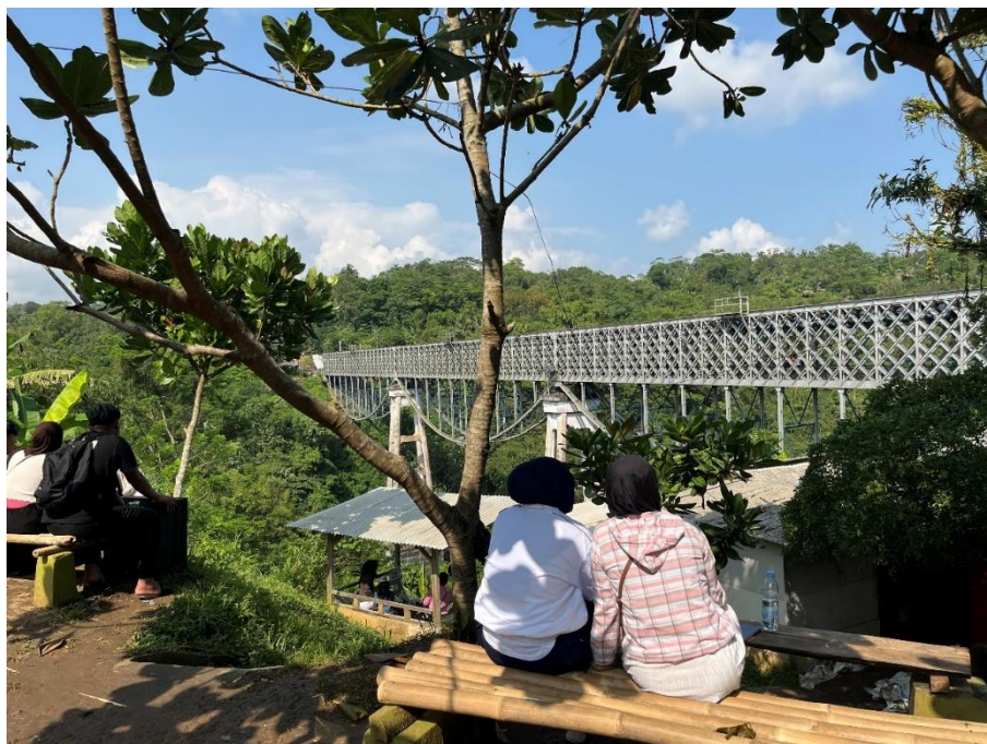
The Cirahong Bridge which connects Ciamis and Tasikmalaya, as a vital object of the Railway Line which was built in 1893 by the Dutch East Indies government. Research Documentation
